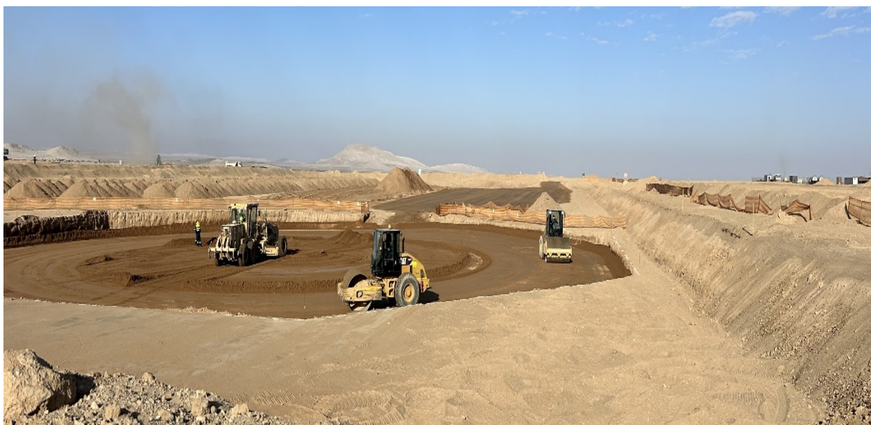
Figure 2: Bulk earthworks for the counter current decantation area at the Tumas Project.
