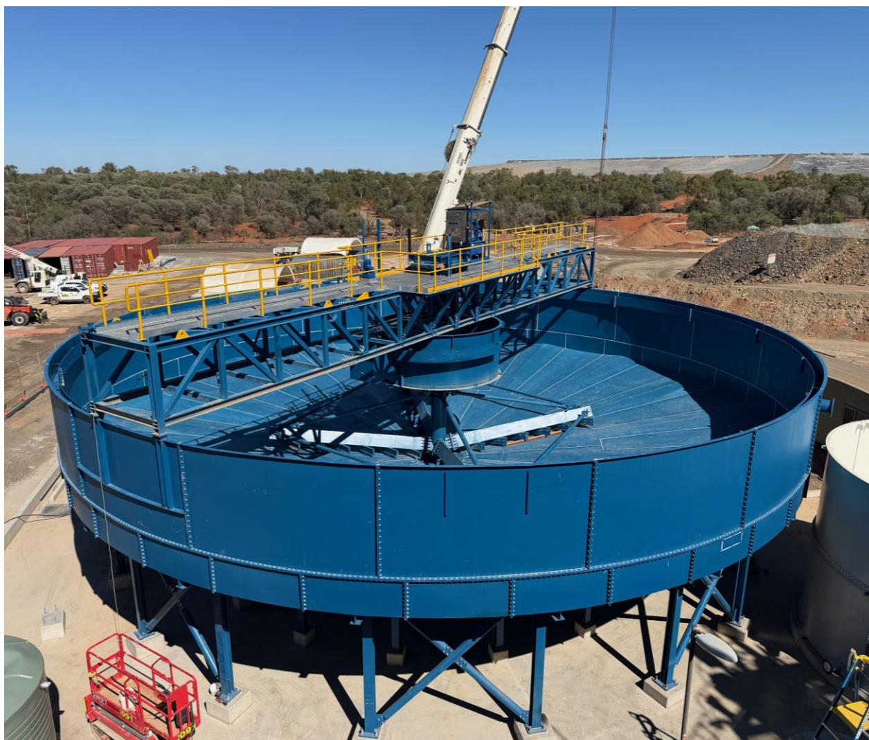
Photo: Tailings Thickener installation at Peak (March 2026)
