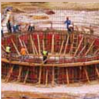
In Construction Kayelekera
