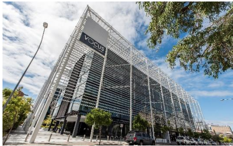
WorkZone West 202 Pier Street, Perth
