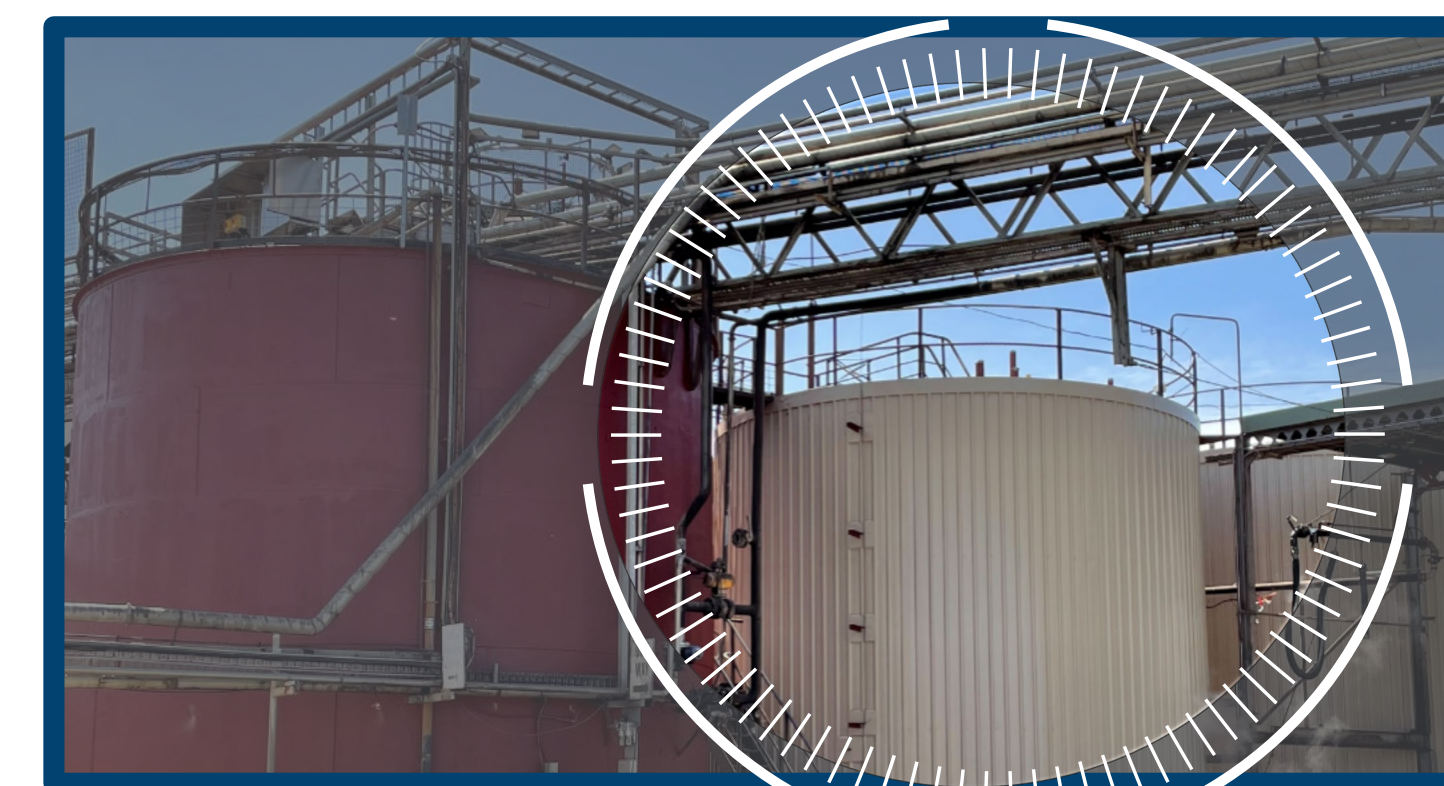
Tank and piping insulation to reduce energy and improve tallow quality.
