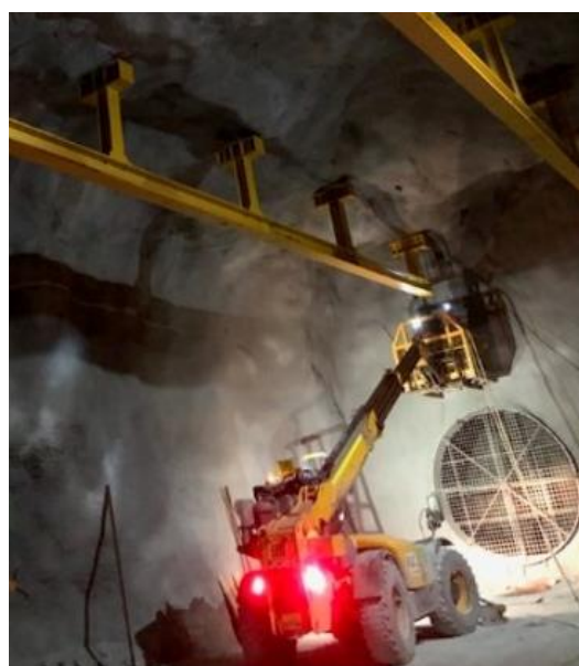
Figure 2: Booster fan chamber construction
